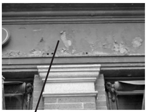
FILL HOLES, CLEAN, PATCH, PREP AND REPAINT EXISTING METAL TRIM BAND
