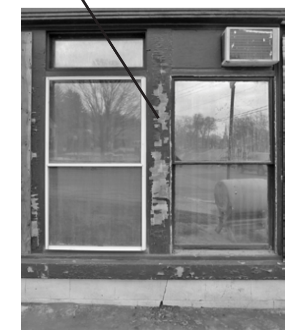
REMOVE LOOSE PAINT, CLEAN PREP AND REPAINT ALL TRIM
