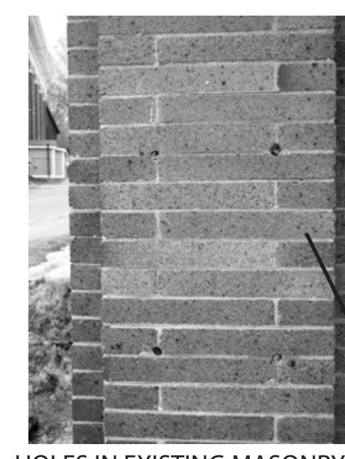
HOLES IN EXISTING MASONRY CORNER TO REMAIN
