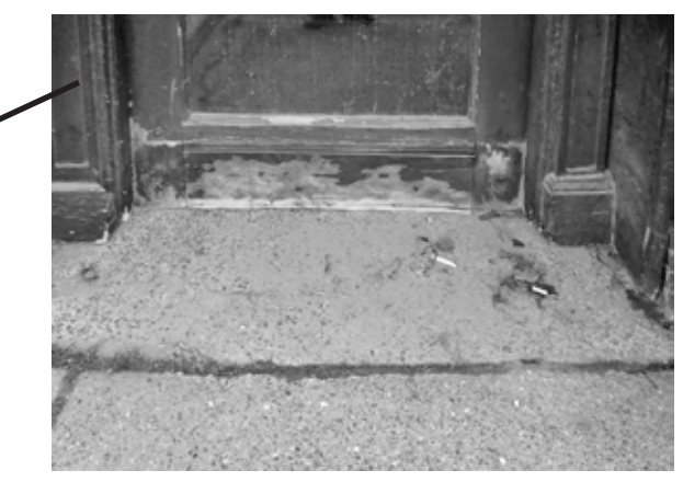
REPAIR DAMAGED BOTTOM SECTION OF EXISTING FRONT DOOR
