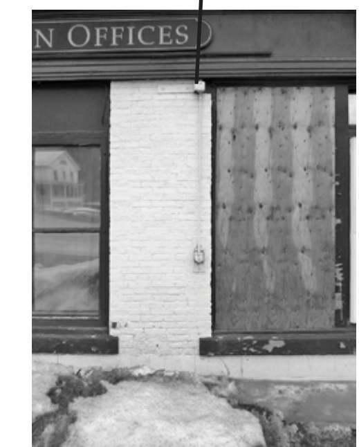
REMOVE & SAVE OLD AWNING HARDWARE - PATCH WALL
