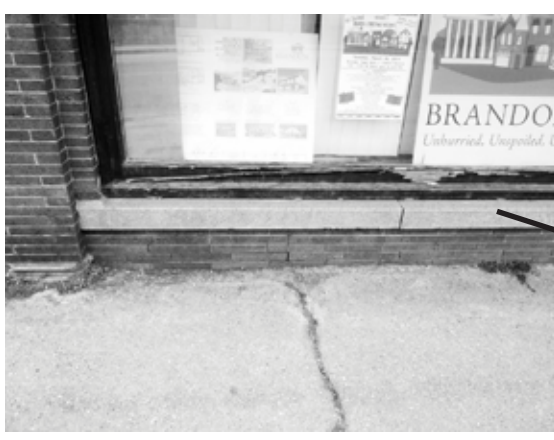
REPAIR DAMAGED WOOD SILL AND PATCH CONCRETE SILL
