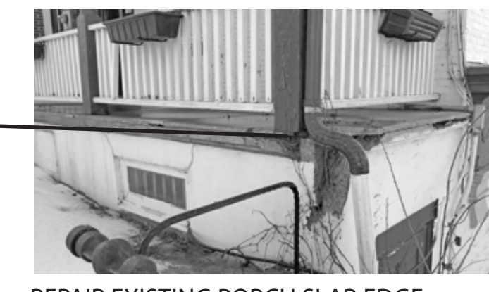
REPAIR EXISTING PORCH SLAB EDGE
