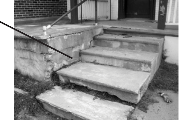
PATCH & REPAIR EXISTING CONCRETE STEPS & WALL
