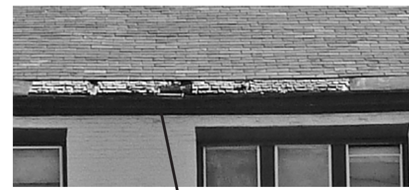
PHOTO OF EXISTING CONDITIONS UNDER TEMPORARY APRON PATCH- REMOVE AND REPLACE ENTIRE APRON AND ADD NEW SHEATHING AS REQ'D.
