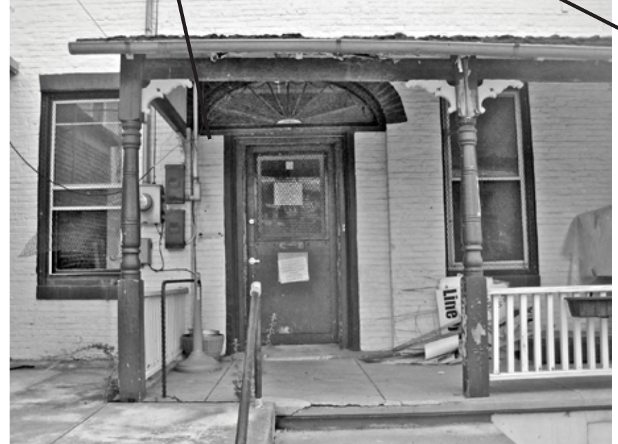
REPAIR PORCH SLAB EDGE - REMOVE GRATING ON DOOR AND REPAIR DOOR FOR SMOOTH OPERATION. REMOVE OLD ELECTRICAL BOXES AND RECONNECT SERVICE TO NEW PANEL
