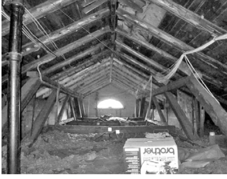
REMOVE ALL OLD WIRING AND OLD INSULATION - CLEAN OUT ALL DEBRIS TO ALLOW INSTALLATION OF NEW INSULATION. STRUCTURAL REINFORCING OF EXISTING RAFTERS TO BE BID AS A DEDUCT ALTERNATE - SEE STRUCTURAL
