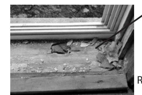
REPLACE ROTTED WOOD WILL TO MATCH EXISTING
