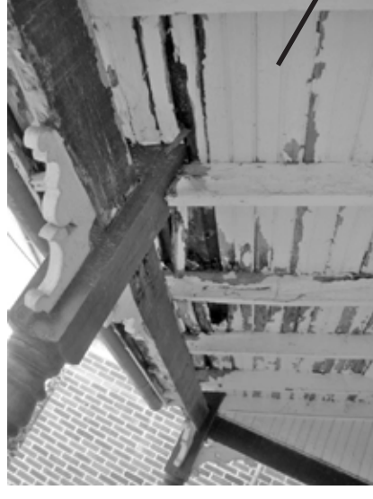
REPLACE PORCH ROOF DECKING (MATCH EXISTG) CLEAN, PREP AND PAINT ALL PORCH DECK, TRIM AND RAILINGS
