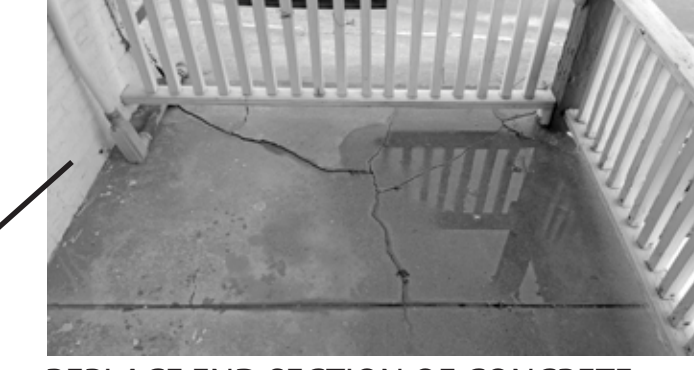
REPLACE END SECTION OF CONCRETE PORCH DECK TOPPING (MATCH EXISTG)
