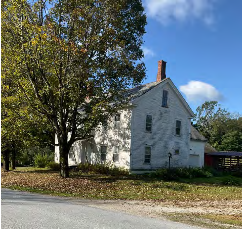
Photograph 1: The former Brandon Town Farm at 1284 Town Farm Road. Camera facing southwest.
