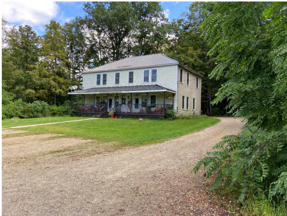
Photograph 22: The Village of Forest Dale, 67 Schoolhouse Road. Camera facing northeast.
