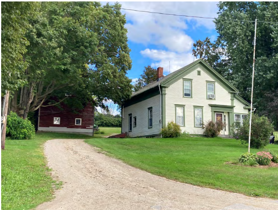
Photograph 42: 1933 Arnold District Road. SR #3. Camera facing east.
