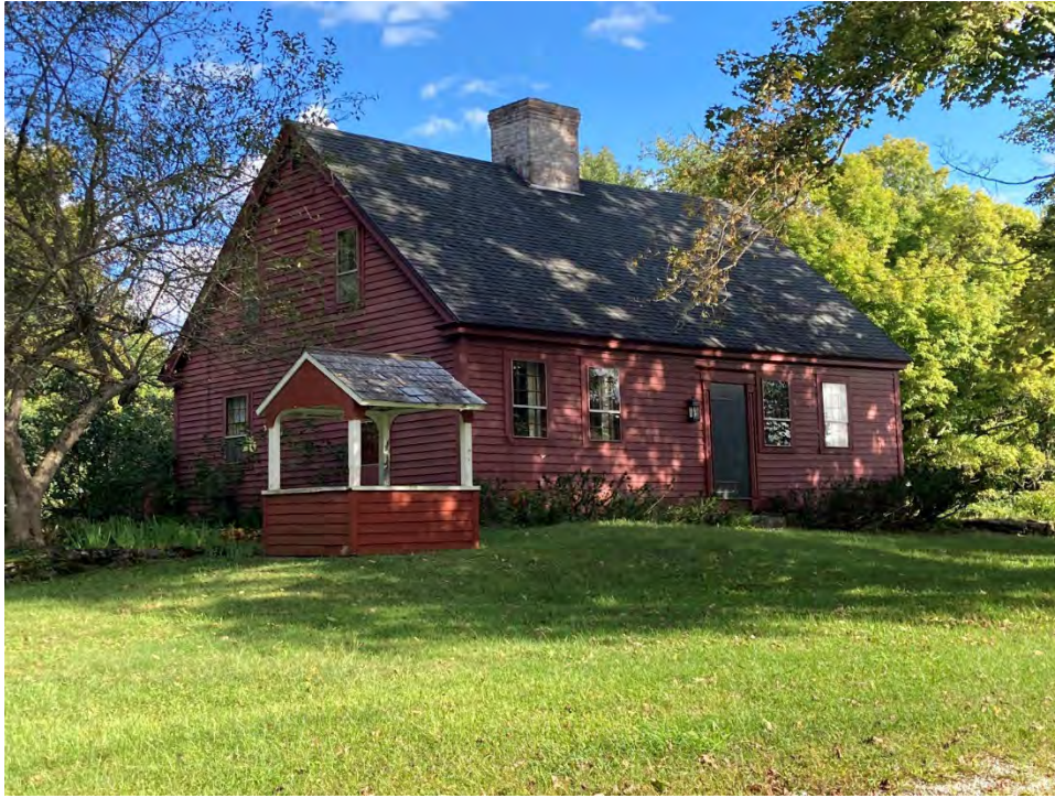
Photograph 43: 927 Hollow Road. SR #7. Camera facing southeast.
