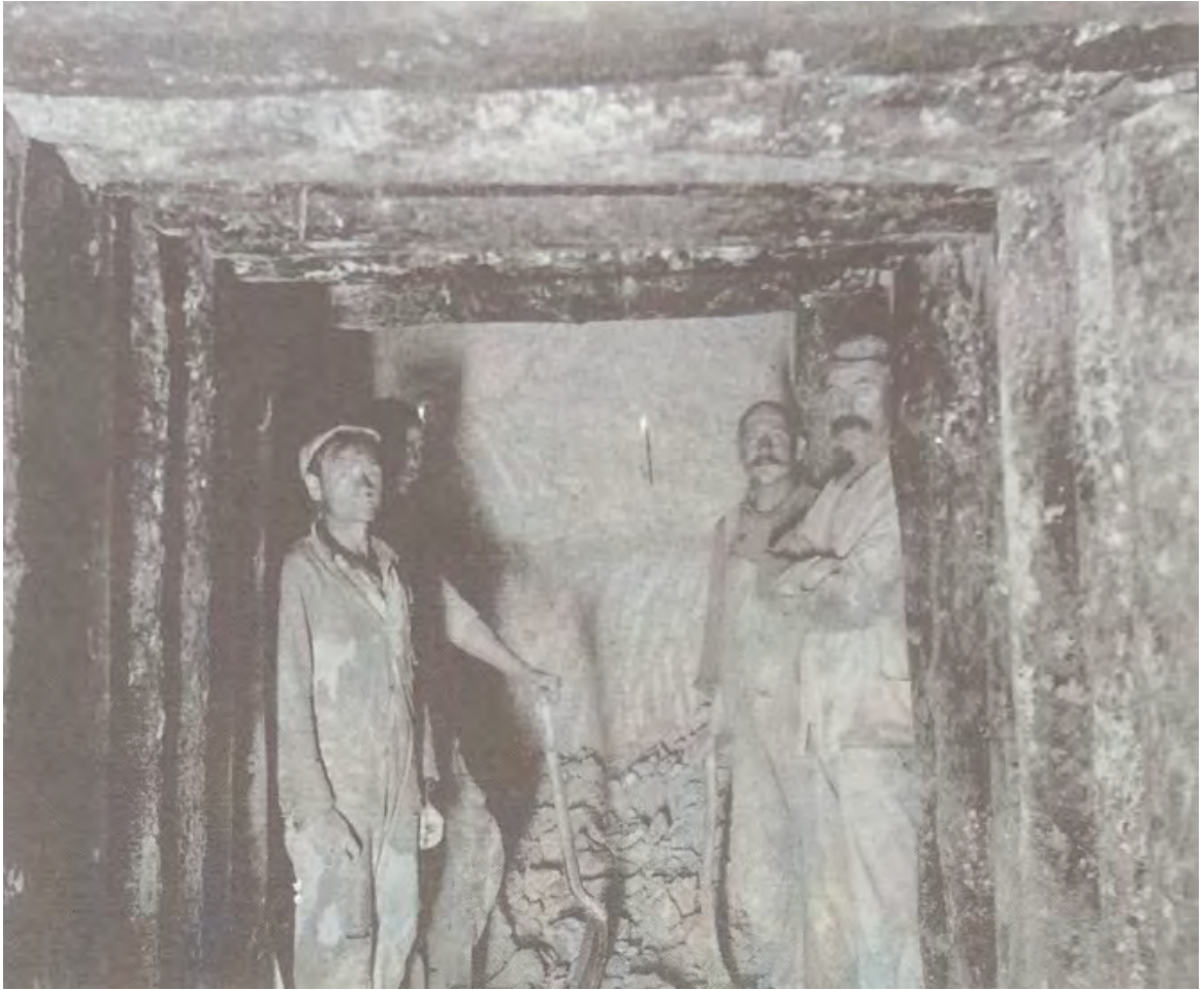
Figure 2: A group of miners extracting Kaolin from a shaft in Forest Dale. Source: Historical Photographs of Brandon and Forest Dale Vermont available at UVM Silver Special Collections Library and Brandon Town Office.
