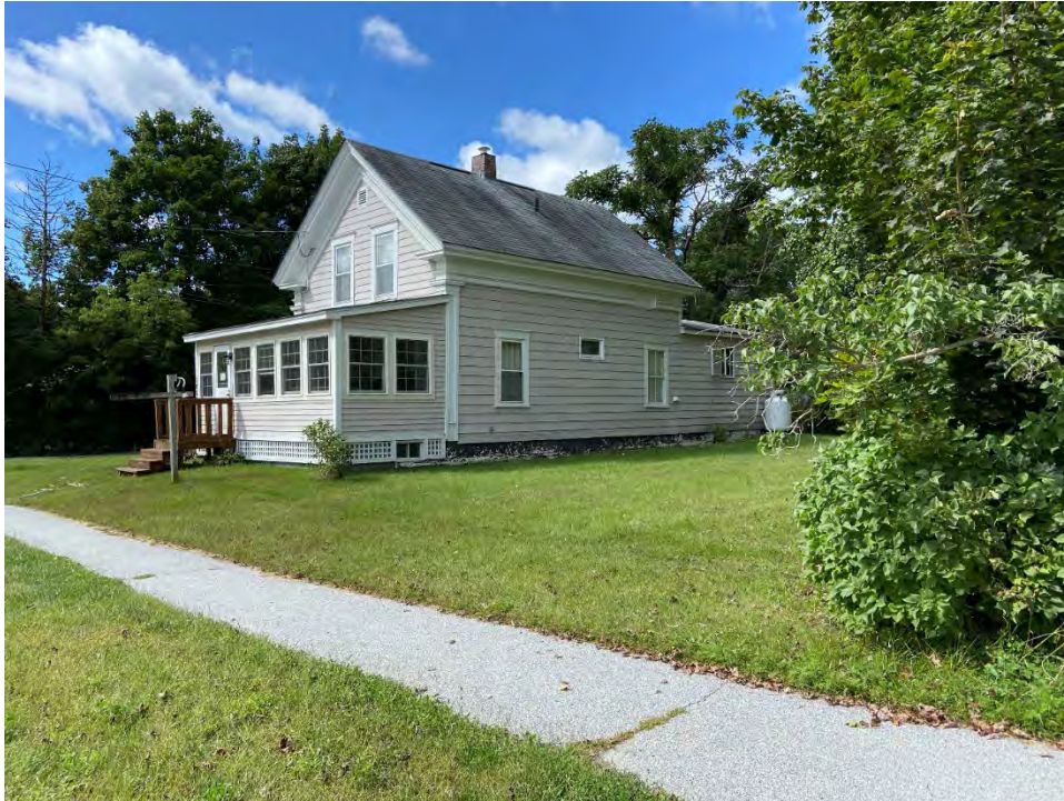
Photograph 37: The Village of Forest Dale, 1820 Forest Dale Road. SR #26. Camera facing southwest.
