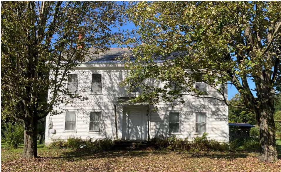
Photograph 3: Façade of the former Brandon Town Farm. Camera facing west.
