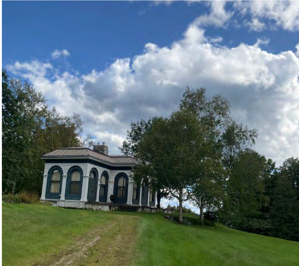
Photograph 5: The Brandon Observatory at 40 Old Farm Road. SR #15 Camera facing northwest.
