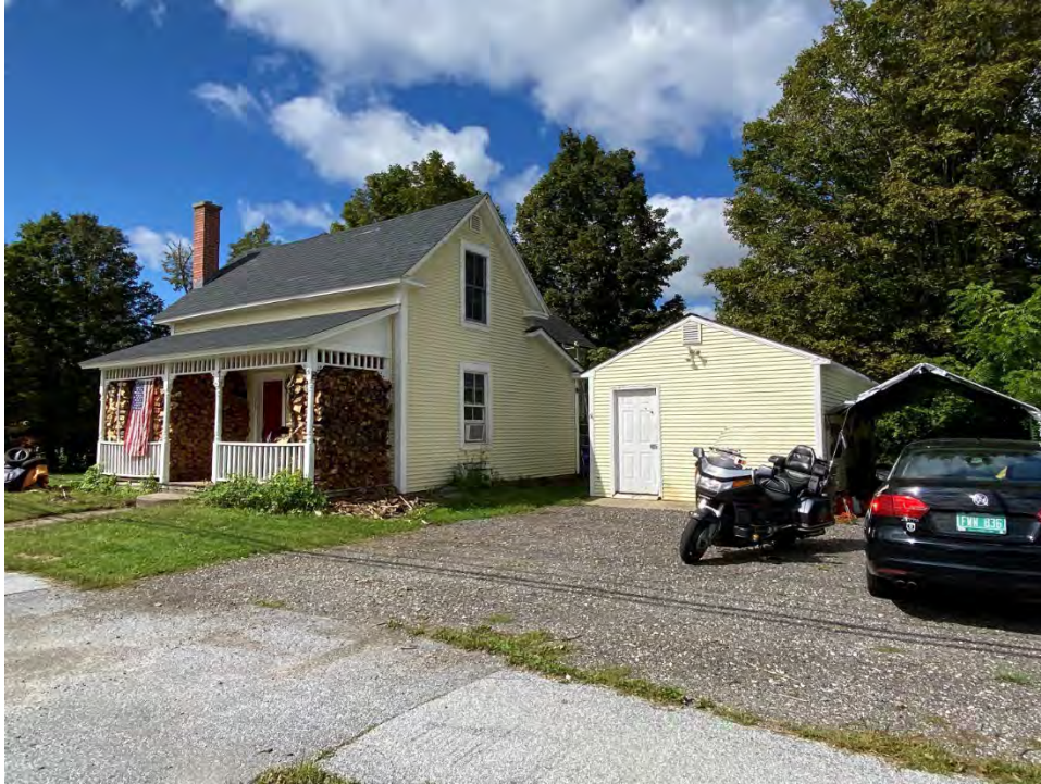
Photograph 35: The Village of Forest Dale, 1920 Forest Dale Road. Camera facing southwest.
