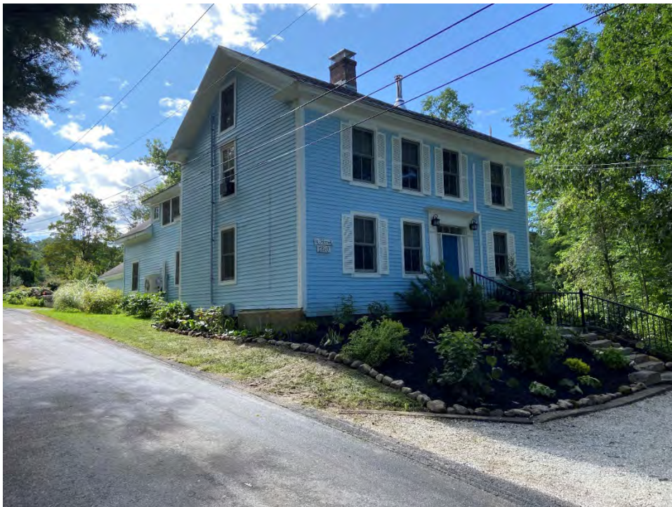
Photograph 14: The Village of Forest Dale, 41 Kennedy Drive. SR #43. Camera facing south.
