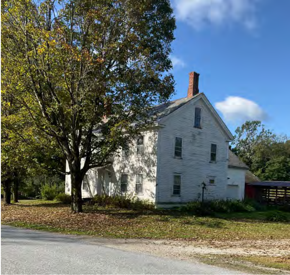
Figure 7: The Brandon Town Farm at 1284 Town Farm Road. Camera facing southwest.
