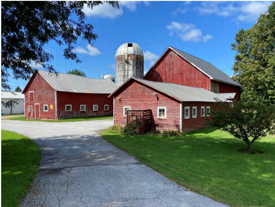
Photograph 24: 2248 Forest Dale Road. Camera facing northwest.
