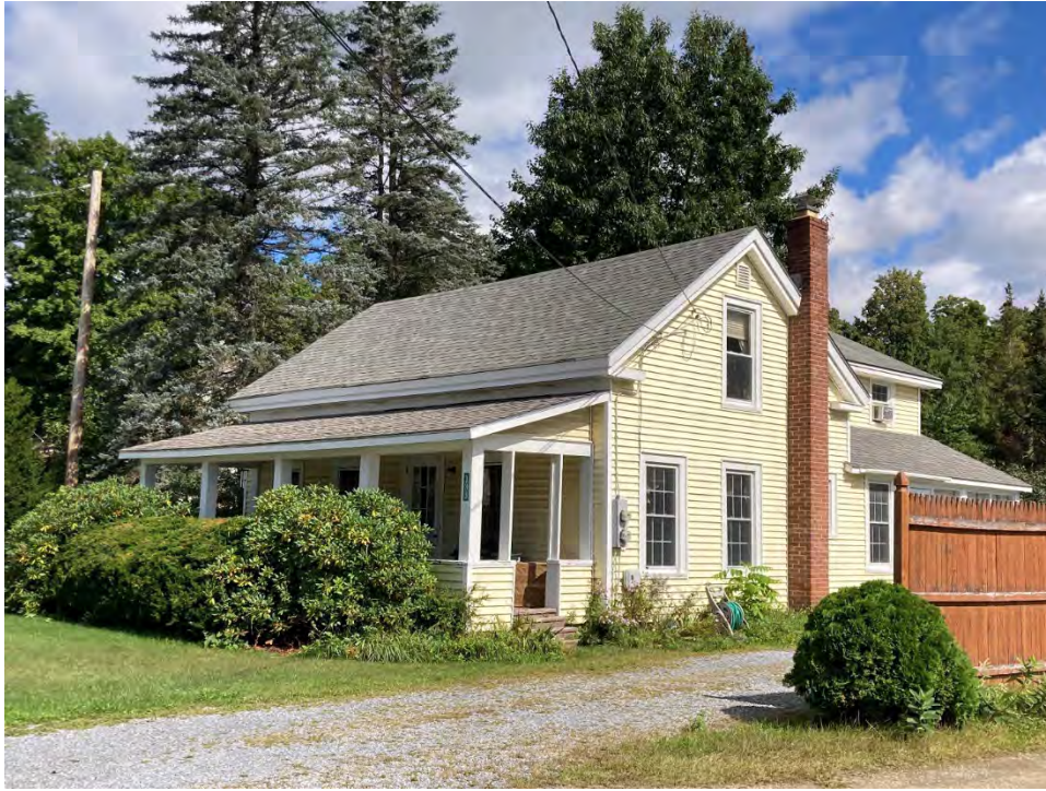
Photograph 27: The Village of Forest Dale, 133 North Street. Camera facing northeast
