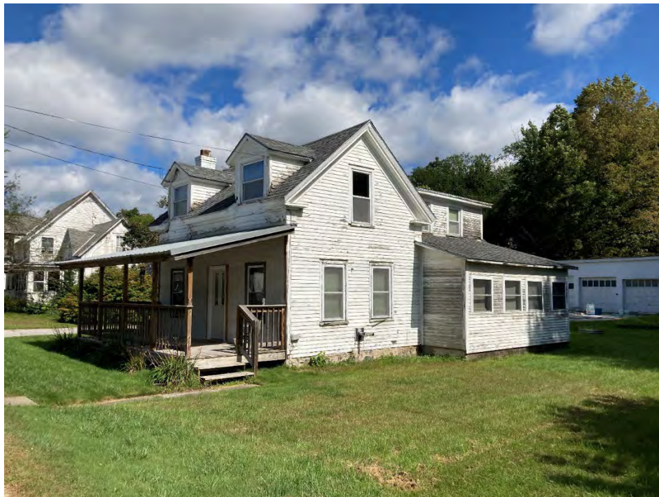
Photograph 26: The Village of Forest Dale, 69 North Street. Camera facing northeast.
