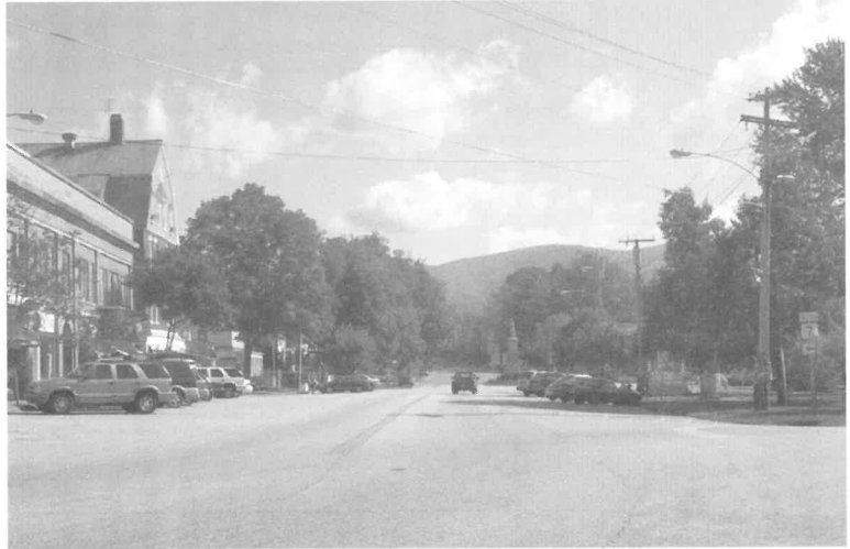
2001 Rte. 7 Rte. 7 is a major intrusion on the historic fabric of the town center. Physically, it bisects the that center, separating the shops on the north side of Central Park from the park itself. Aesthetically, it is an excessively wide no-man's-land of uninviting asphalt.
