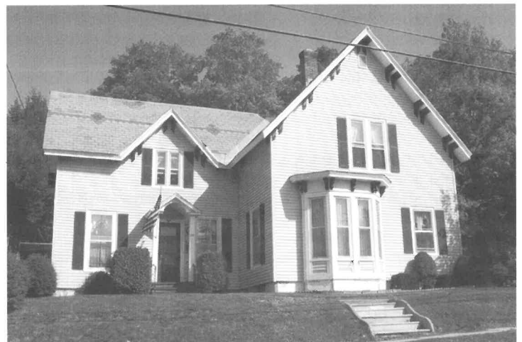
To simplify the installation of vinyl or aluminum siding, original wood details are often removed. As in this example, a building's character may be significantly changed.
