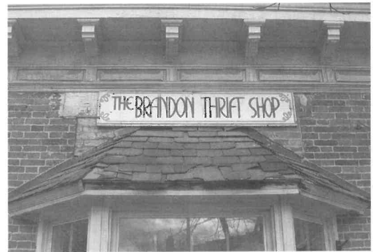
2001 Sign Signs should be designed for a specific location. This sign should have been longer, to cover the wall patch.
