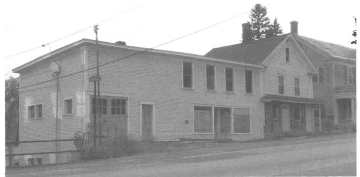
2001 Former Sunoco Station, 12-14 Conant Square
