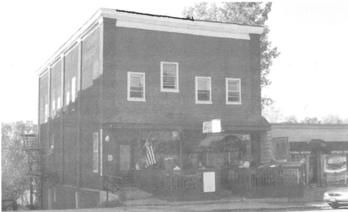
This building certainly looked better with its original windows.
