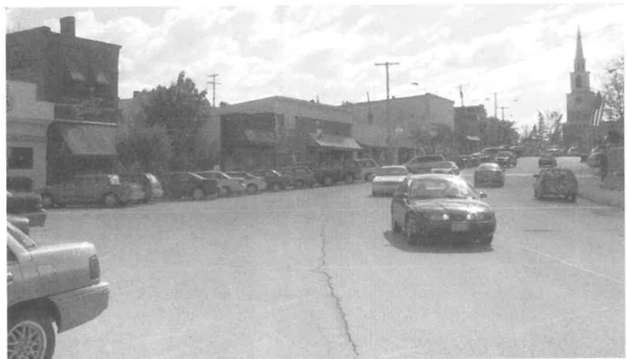
LOCATION 3.2 Looking south along Center Street. The street is wider than necessary. A green space could be added in front of Buildings Nos. 25 and 26.
