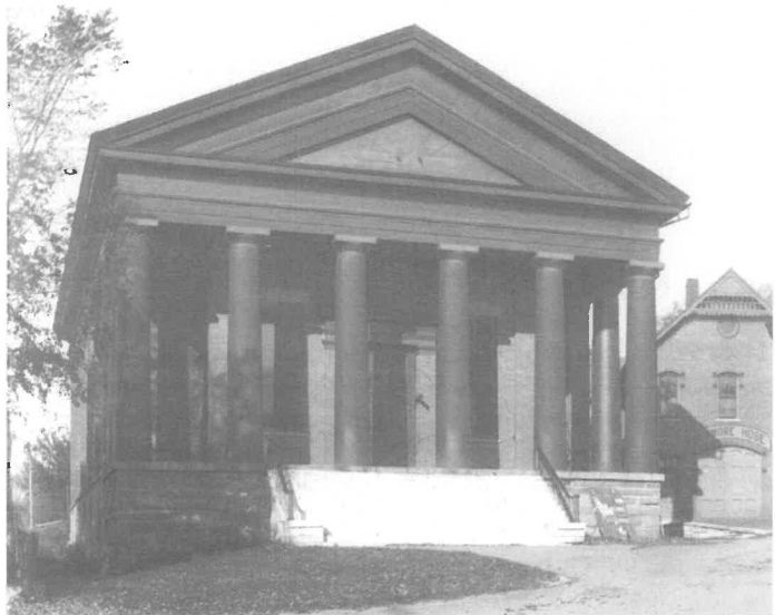
1900 Town Hall Note the brown and beige Victorian color scheme and the front steps. These are the second set of steps. The original steps were slightly wider with piers at each end and in the center which lined up with each of the four center columns. The present steps are the third set.
