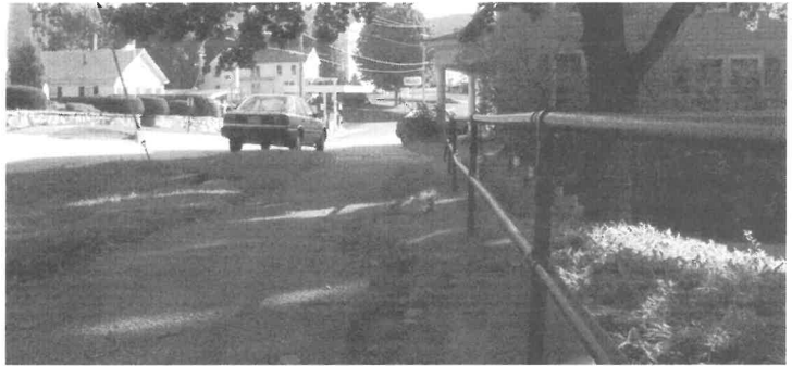
LOCATION 2.4 Toward the eastern end of Conant Square the sidewalk turns to align with the Town Hall. The view is excellent, but the walk soon disappears into the street.
