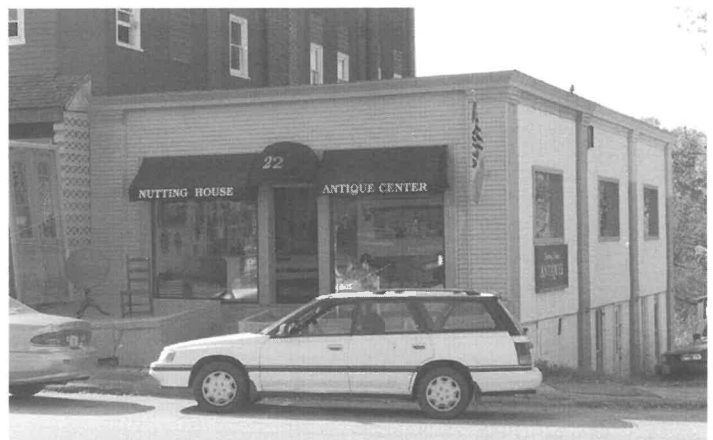
2001 Commercial Bldg. (Nutting House Antique Center), Center Street
