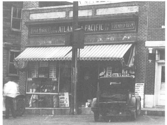
1930 Atlantic and Pacific Note how the A&P sign fits into the designated sign band in the building's parapet.
