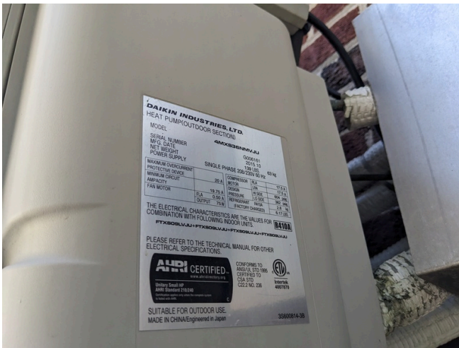
Condenser 2N by Daikin; Model: 4MXS36NMVJU
