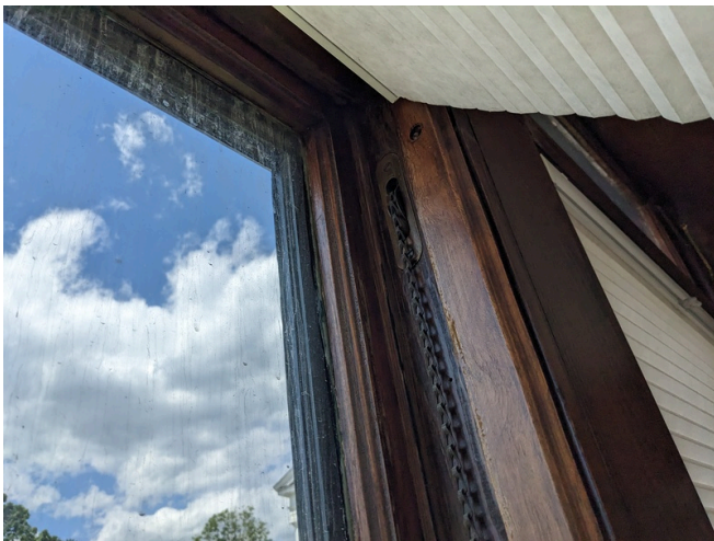
First Story West Window
