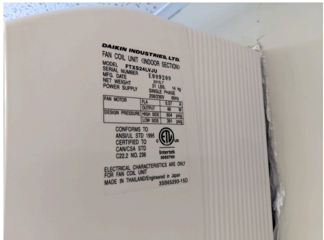
Evaporator by Daikin; Model: FTXS24LVJU
