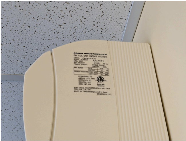
Evaporator by Daikin; Model: FTXS12LVJU
