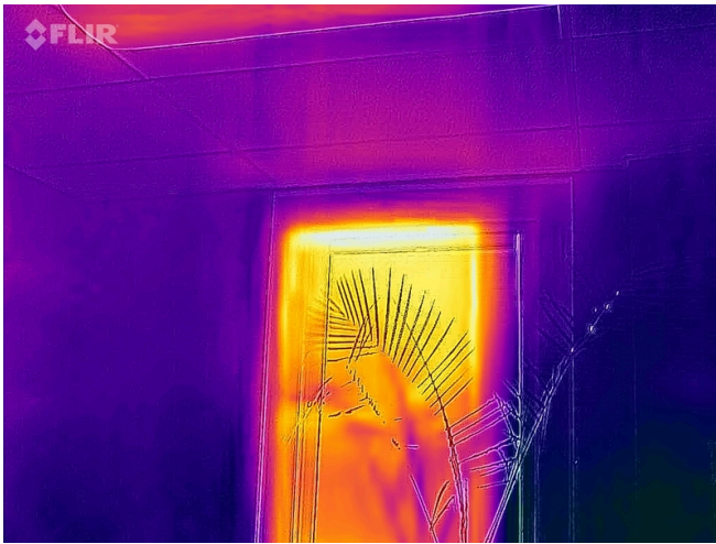
IR Second Story South Wall Window
