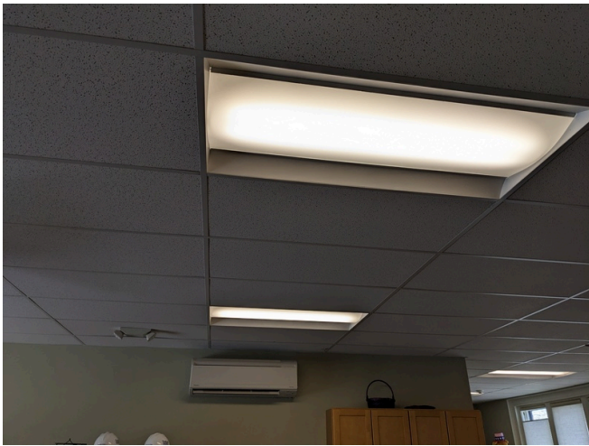
Lighting in the Second Story Lobby
