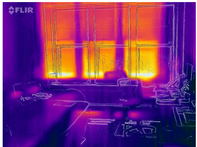
IR Second Story South Wall Windows
