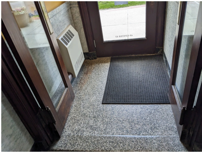
First Story Glass Door in the Clerks Office
