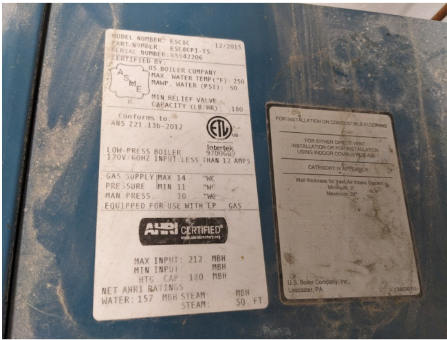
Hydronic Boiler by US Boiler Company; Model: ESC8C
