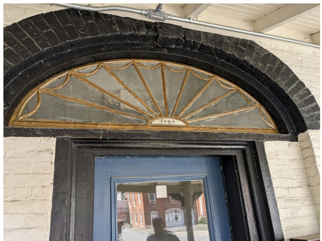
North Entry to the Upstairs Town Managers Office Fan Window
