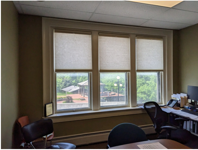
Second Story South Wall Windows
