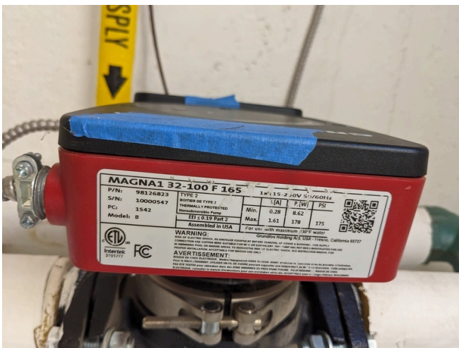
178 W (1/4 HP) Pump by Grundfos; Model: B; MAGNA1 32-100 F 165;
