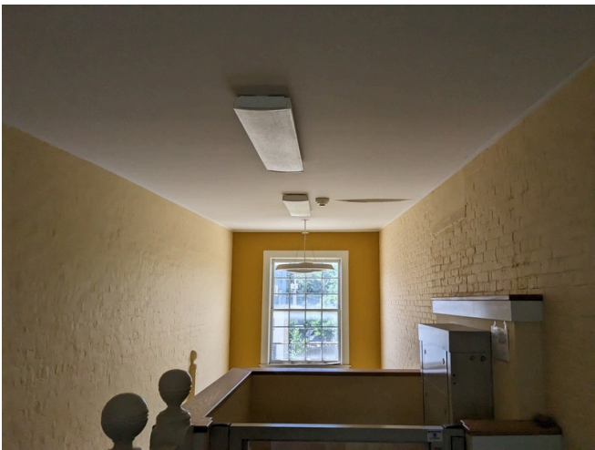
Lighting and South Wall Window in the Second Story of the Shared Entry Stairway with Wheelchair Lift
