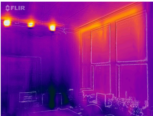
IR First Story East Wall Windows
