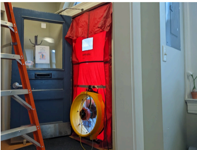
Blower Door Setup Second Story with Stairway
