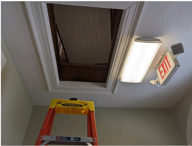
Attic Access in the North Entry Foyer
