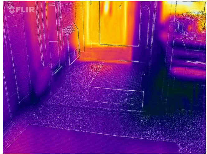
IR First Story South Entry Foyer Outside Door
