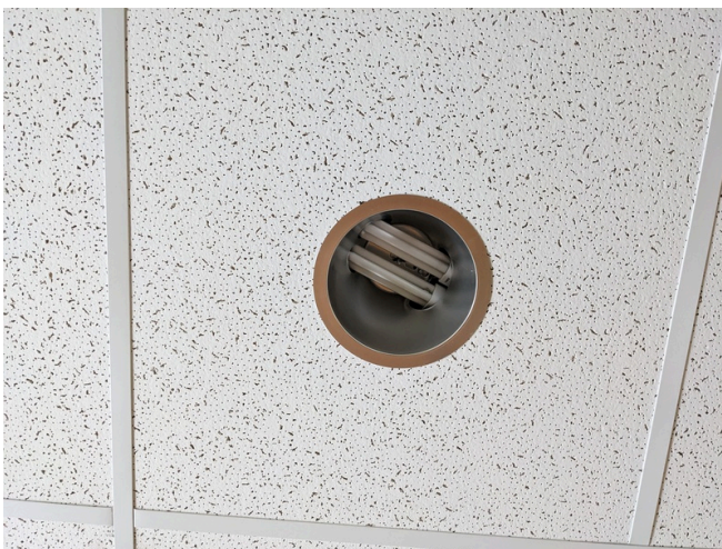
CFL Recessed Can Lighting
