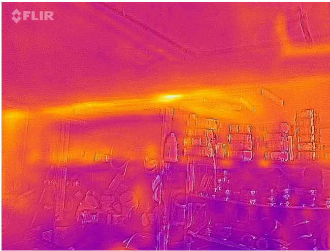
Building 5 - Interior IR - Ceilings and Walls
