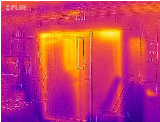
Building 2 - Interior IR - Entry Doors
