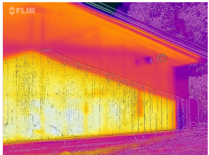
Building 5 - Exterior IR - Southern Elevation
