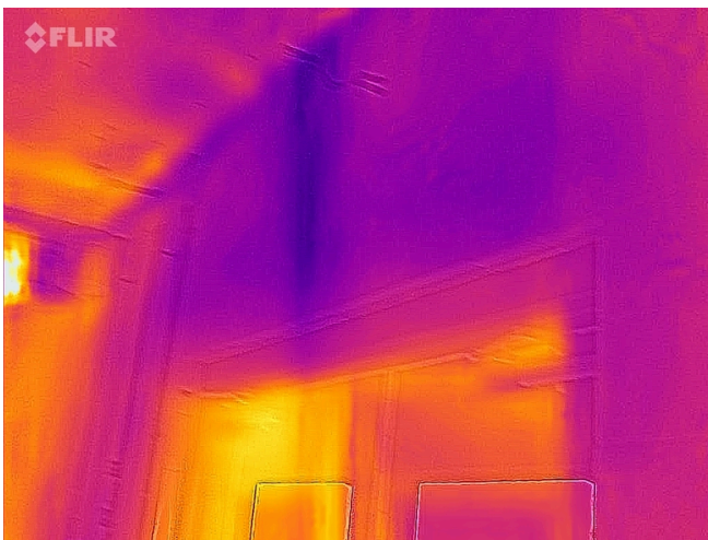
Building 3 - Interior IR - Ceiling Line
