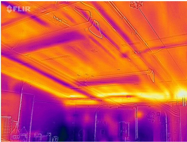
Building 1 - Interior IR - Vaulted Ceiling
