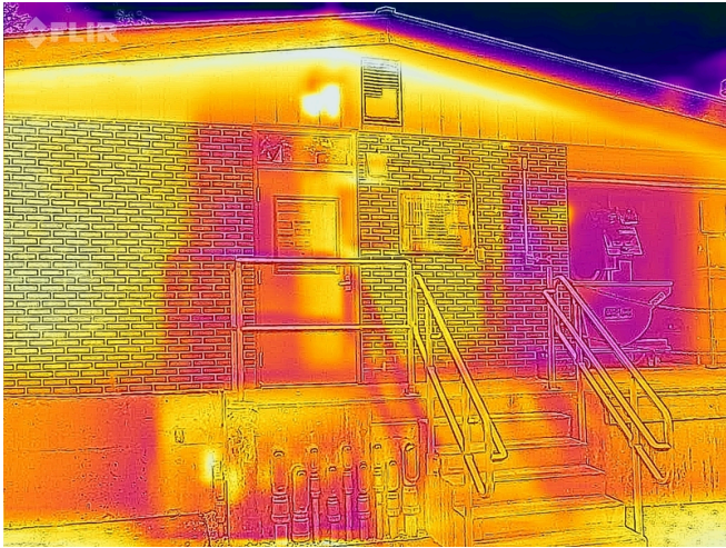
Building 2 - Exterior IR - Eastern Elevation
