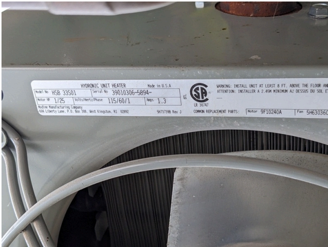
Hydronic Heater by Modine; Model: HSB 33S01
