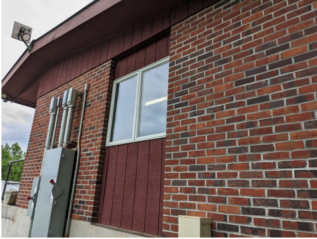
B2 West Wall Window
