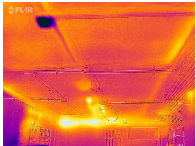
Building 2 - Interior IR - Ceiling
