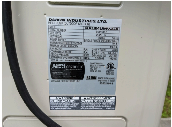
ASHP Condenser by Daikin; Model: RXL24UMVJUA
