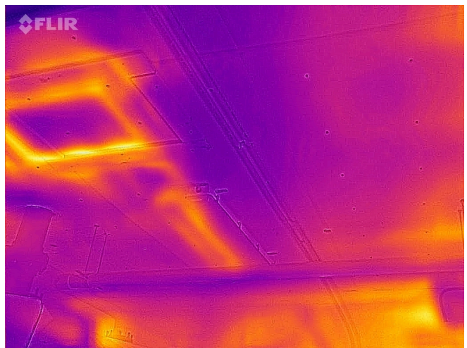
Building 3 - Interior IR - Ceiling
