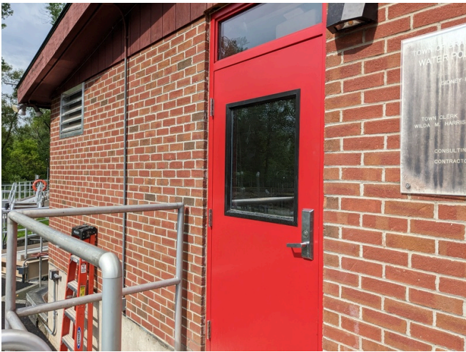
B2 East Wall Main Entry Door
