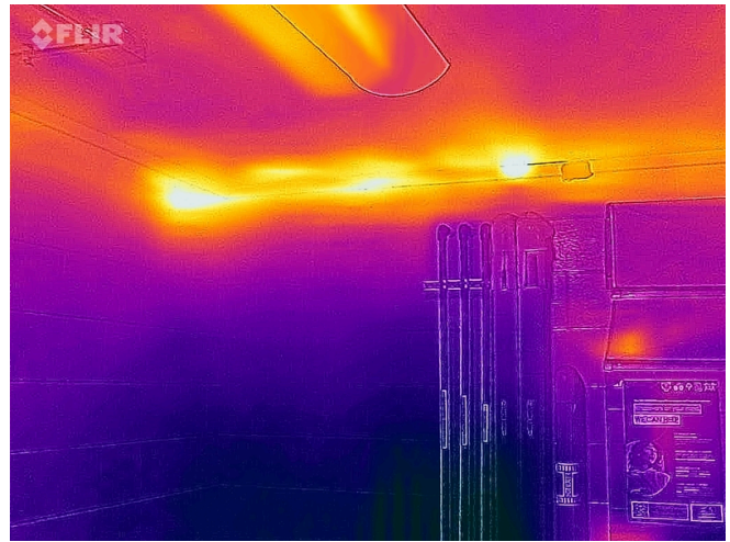
Building 2 - Interior IR - Ceiling Line
