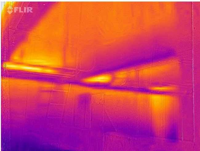
Building 1 - Interior IR - Basement Vault
