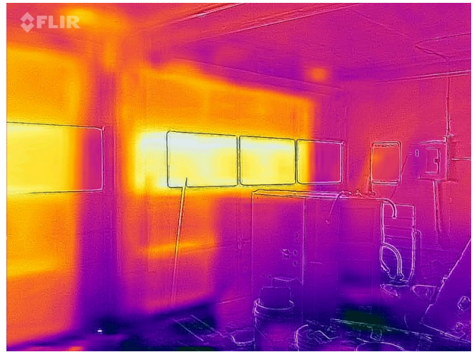
Building 5 - Interior IR - Overhead Doors
