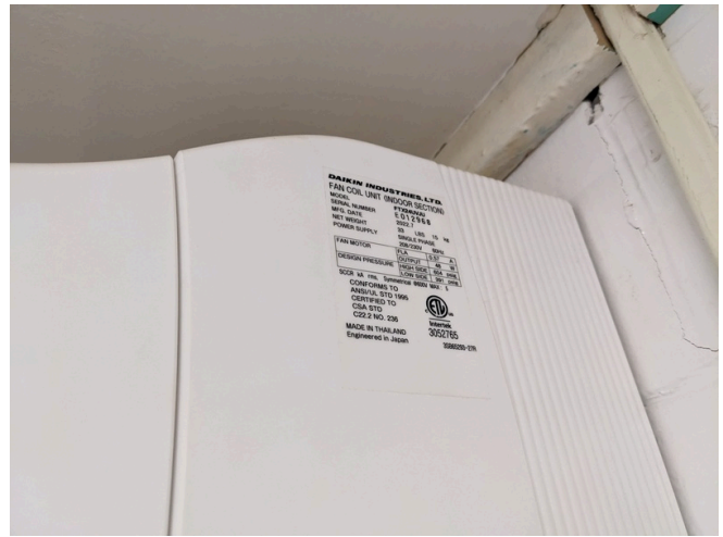
ASHP Evaporator by Daikin; Model: FTX24UVJU
