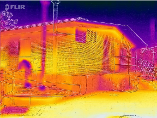
Building 2 - Exterior IR - Southern and Eastern Elevation
