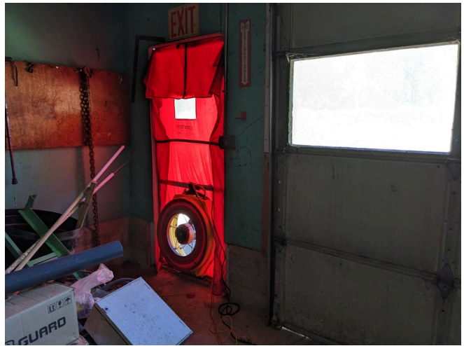
Building 5 - Blower Door Setup
