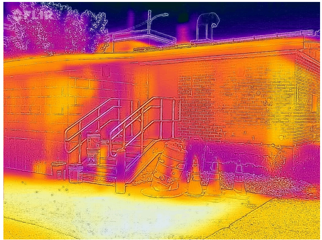
Building 1 - Exterior IR - Northern Elevation
