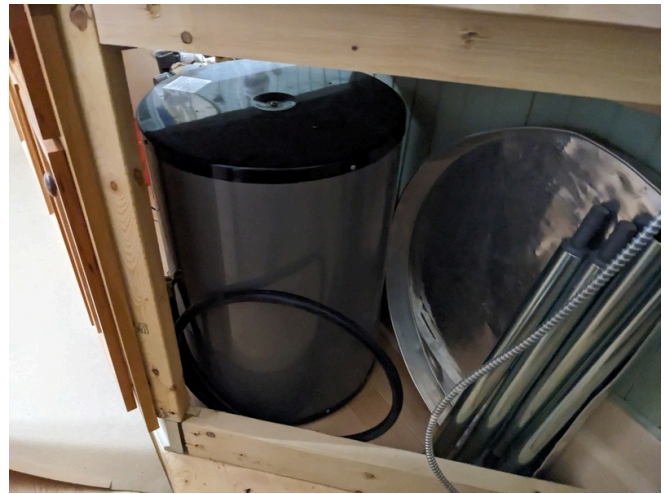
Small DHW in the Second Story Concession Kitchen
