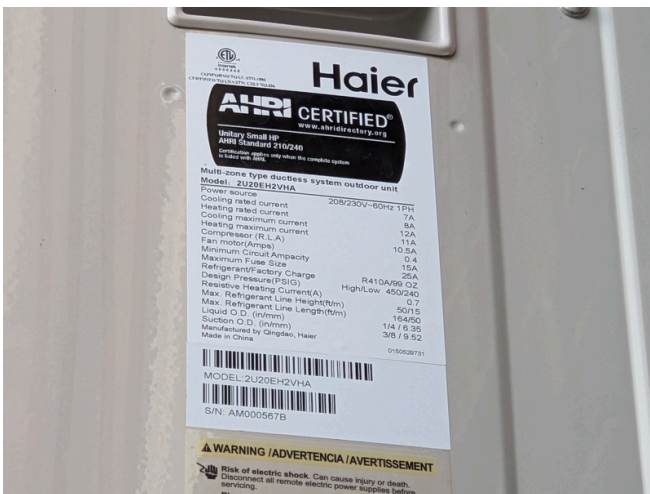
Multi Split ASHP Condenser by Haier; Model 2U20EH2VHA
