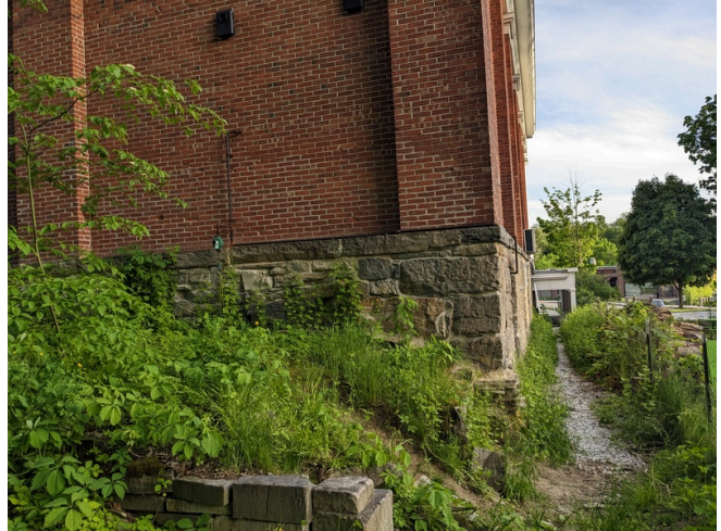
Northwest Corner Stone Foundation
