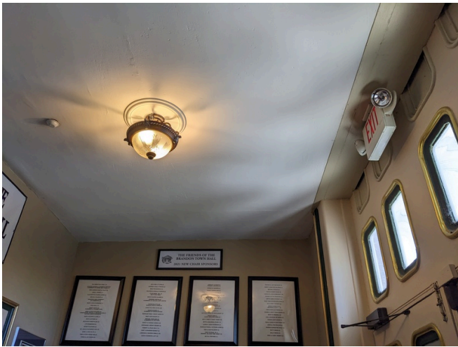
Second Story Front Entry Foyer
