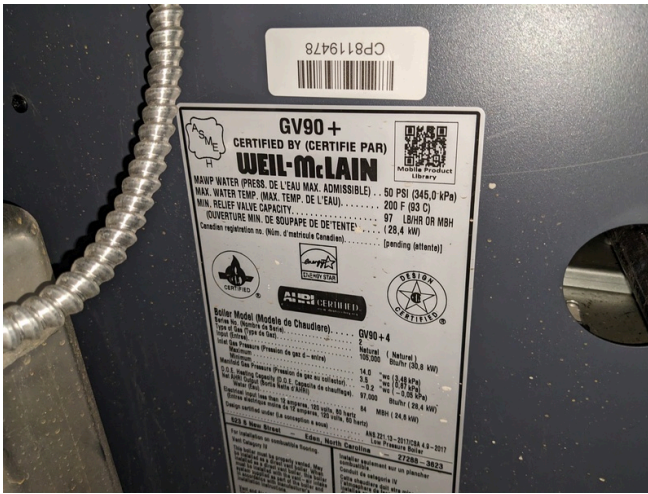
Hydronic Boiler by Weil McLain; Models 90+4
