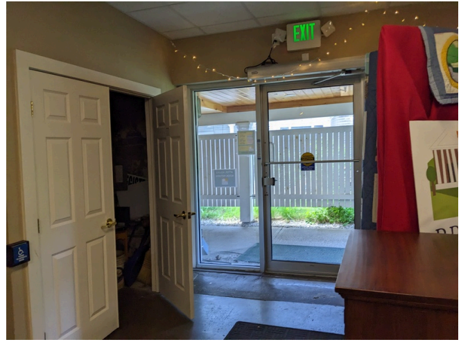
First Story West Side is the Main Entry to the Lower Hall; Entry Closet with Electrical Service Panel
