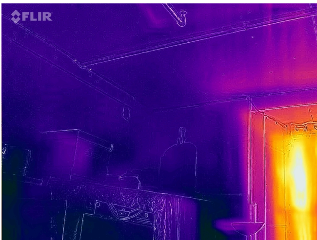
IR First Story West Wall and Window
