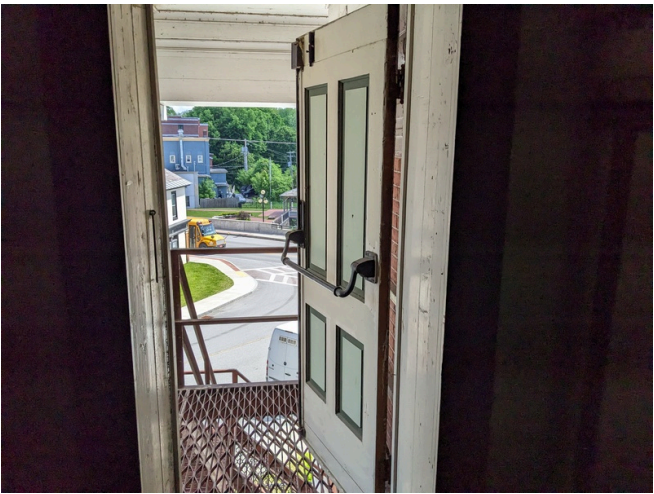
Second Story Balcony Emergency Exit Door to the Metal Exterior Stairs
