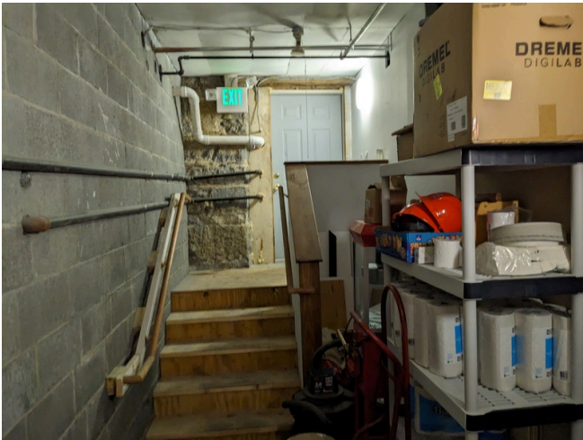
First Story West Back Exit Door
