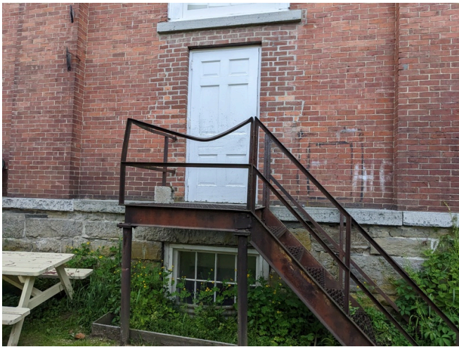
East Wall Theater Back Stage Exit
