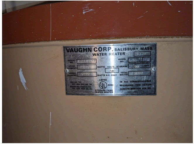
New - DHW by Vaughn Corp; Model C-30; 30 gallon
