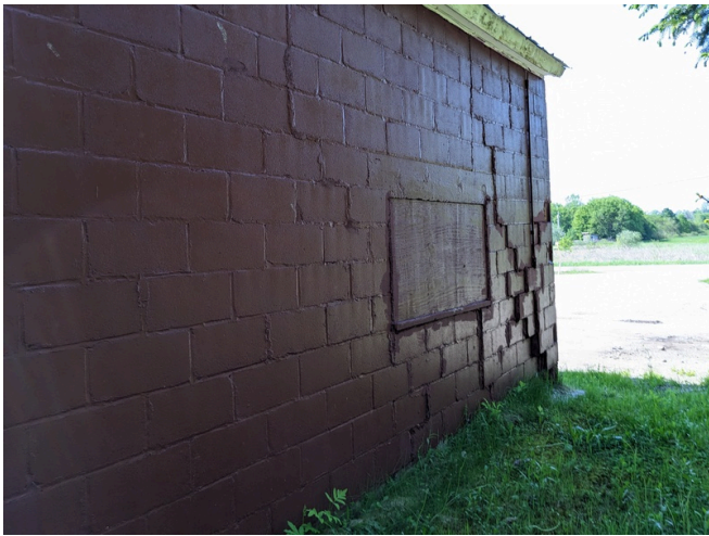
Old - East Wall
