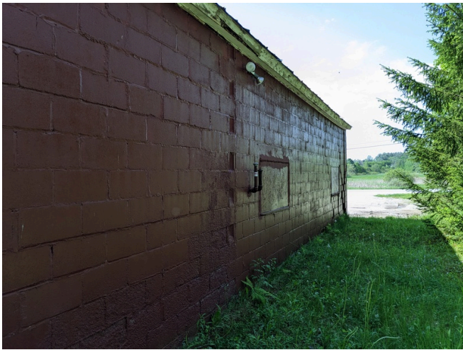
Old - East Wall
