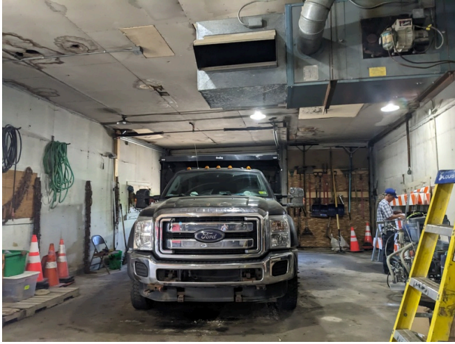
Old - Looking North
