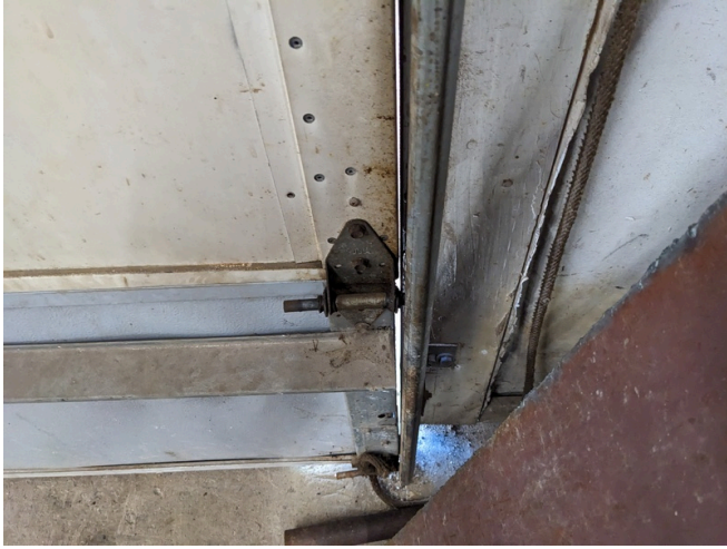
New - Draft Around Overhead Door
