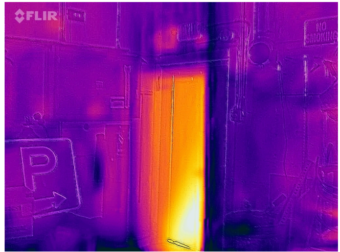
New - IR Southeast Corner Entry Door
