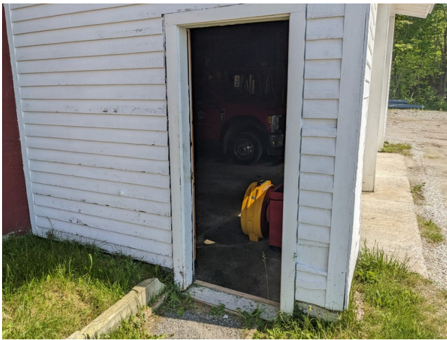
Old - Entry Door on the North Wall
