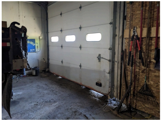
Old - North Wall Overhead Door
