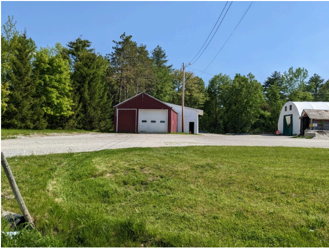
Old Building, Elevation North
