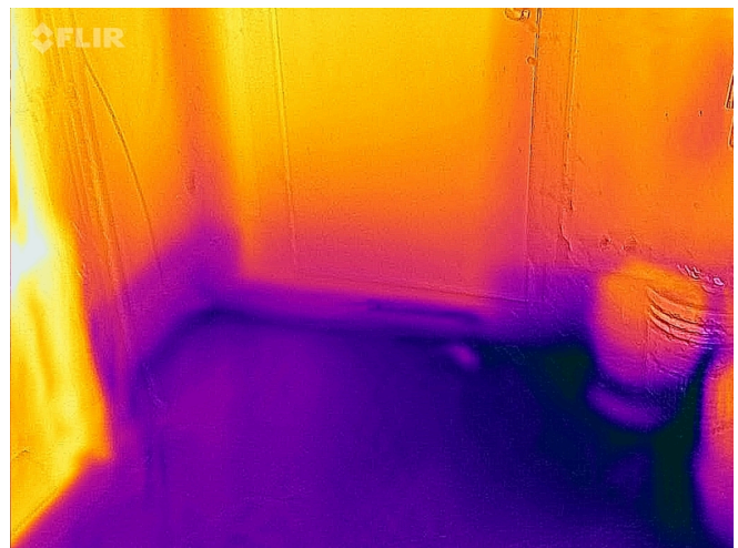
Old - IR North Wall Entry Door and Floor
