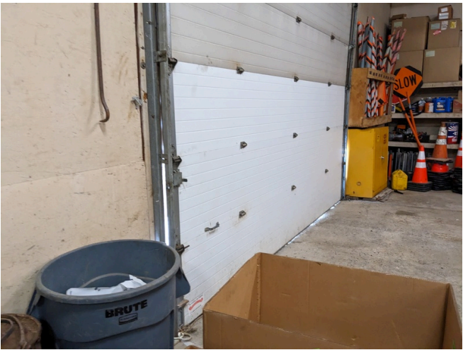
New - Draft Around Overhead Door
