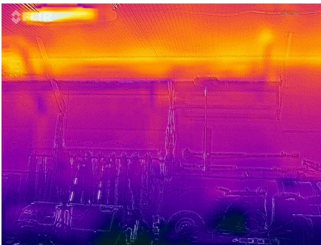
New - IR North Wall in the West Room
