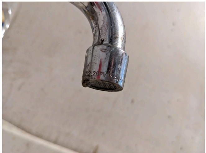
New - 2.2 GPM Rated Flow at the One Faucet
