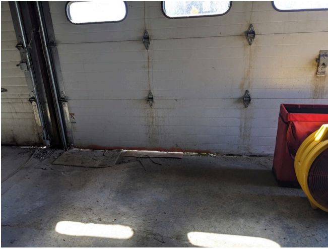
Old - West Wall Overhead Doors
