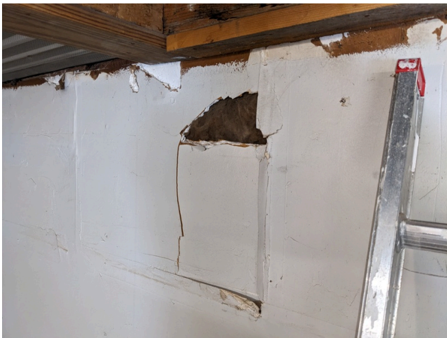
New - Wall Insulation
