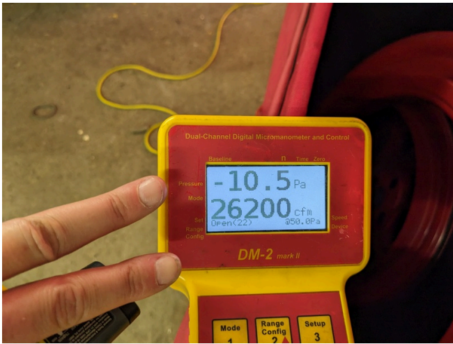
Final New Building Both Room Cannot Depressurize
