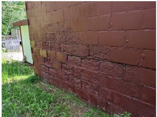
Old - East Wall CMU block
