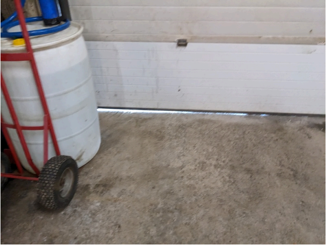
New - Draft Under the South Overhead Door
