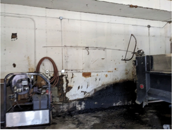
Old - East Wall
