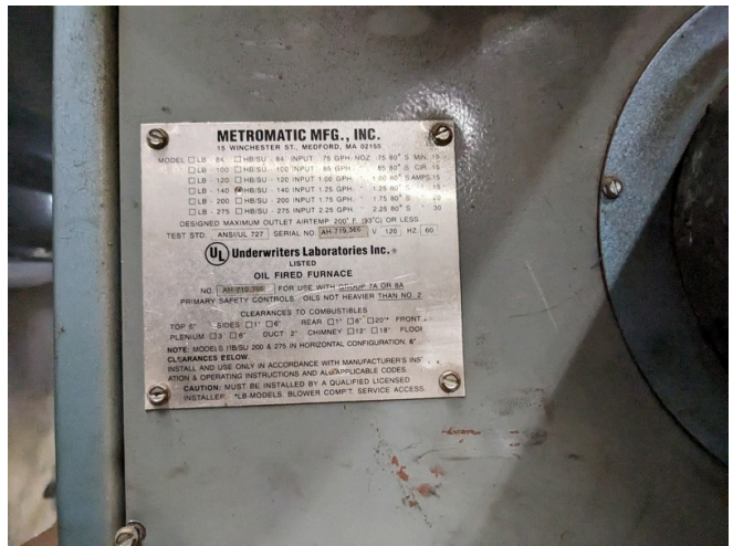
Old - Furnace by Metromatic MFG; Model HB/SU-140; 1.25 GPH
